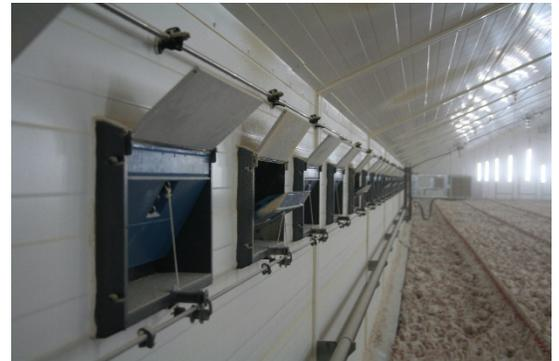
Photo: Cobb Vantress Inc: "Air Inlets in a house"
