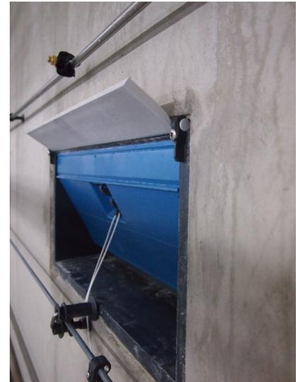
Photo: Cobb Vantress Inc: "Air Inlet in a house"
