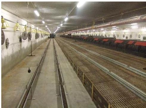
*Photo 2 (left): In production, 4 rows of LED lamps in 14 m wide house should be positioned over the scratch area and at the end of the slats and no lights directly above or shining into the nests.*
